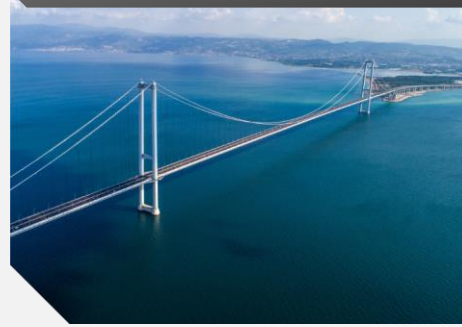
GEBZE - ORHANGAZI - İZMİR MOTORWAY
