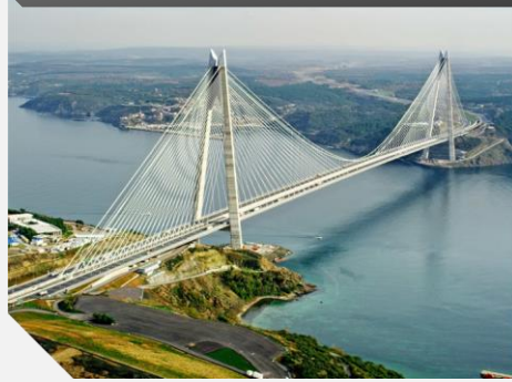
YAVUZ SULTAN SELİM BRIDGE
