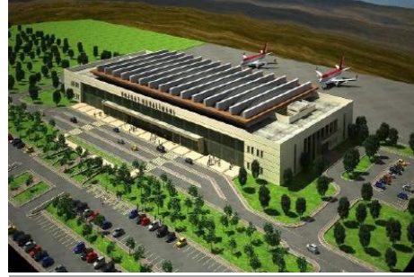
YOZGAT AIRPORT (EPC) 2 MIL. PASS/YEAR 2025
